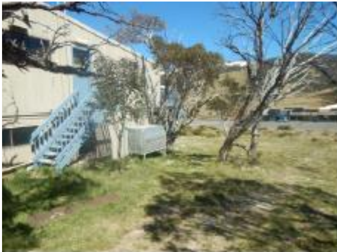
Figure 5. Northern view of the lodge
