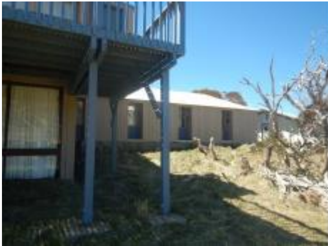
Figure 8. Western elevation of lodge
