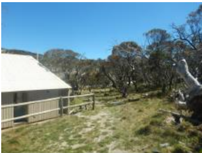
Figure 9. View of rear of lodge, toward entrance path
