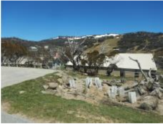
Figure 4. Eastern view of the lodge with carpark to the left
