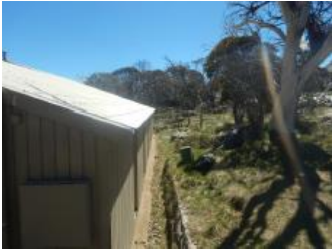
Figure 7. Eastern view of the lodge (boundary at retaining wall)
